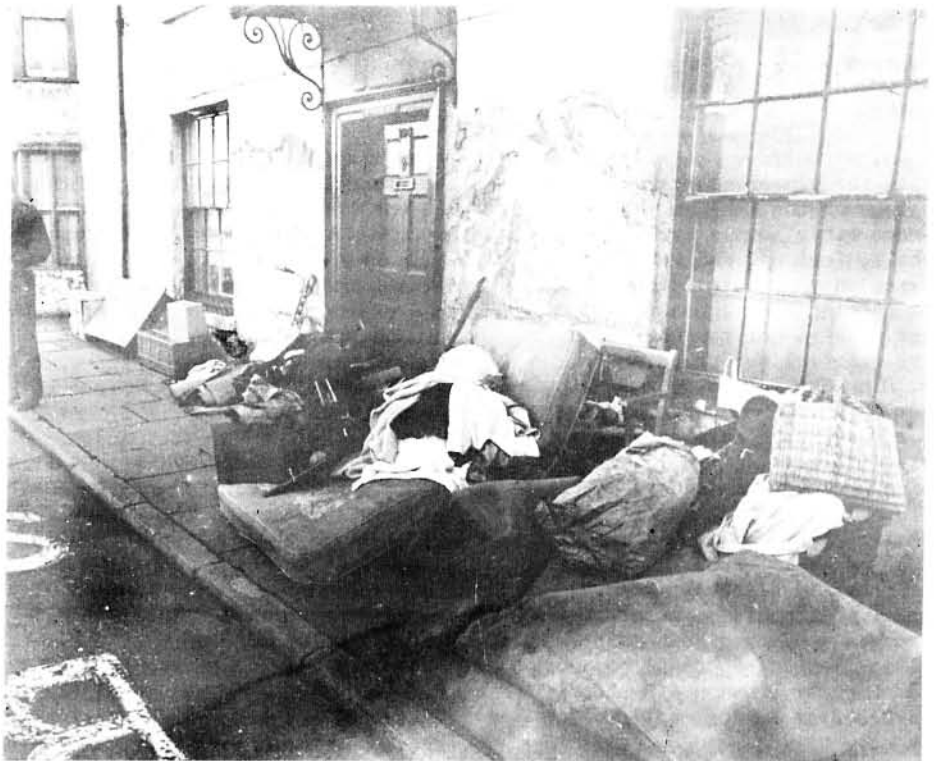
Squatters belongings piled outside. (Photo. John Beeching)
